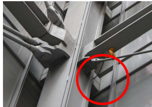
Figure 1- 'Dog-leg' penetrating building envelope
