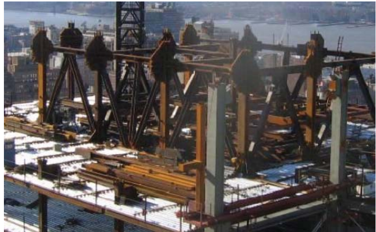
Figure 11: Core bracing during construction, courtesy of Thornton Tomasetti
